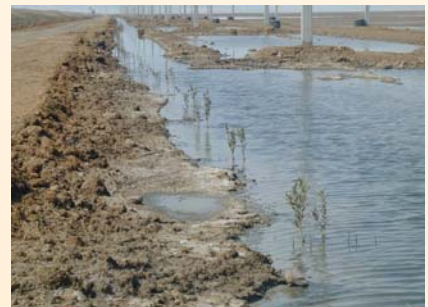
The drainage canal to the sea.
